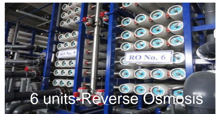
The first state-of-the-art water treatment plant in the Philippines that taps into Laguna Lake which uses microfiltration and reverse osmosis filtration method.
